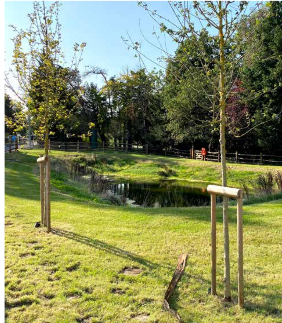
Landscaped attenuation basin
