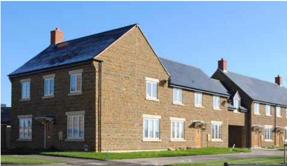
John Harper Road, Adderbury, arrangement of different house types to create a corner and continuous frontage with archway to rear parking court
