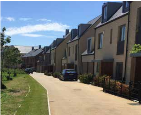
Shared surface lane providing access to properties
